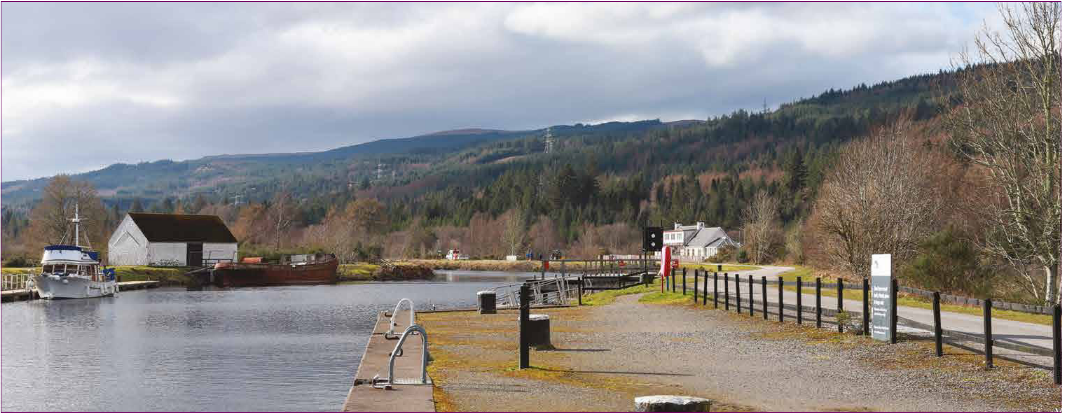
Viewpoint 10: Caledonian Canal Boat Lift (Existing view)
