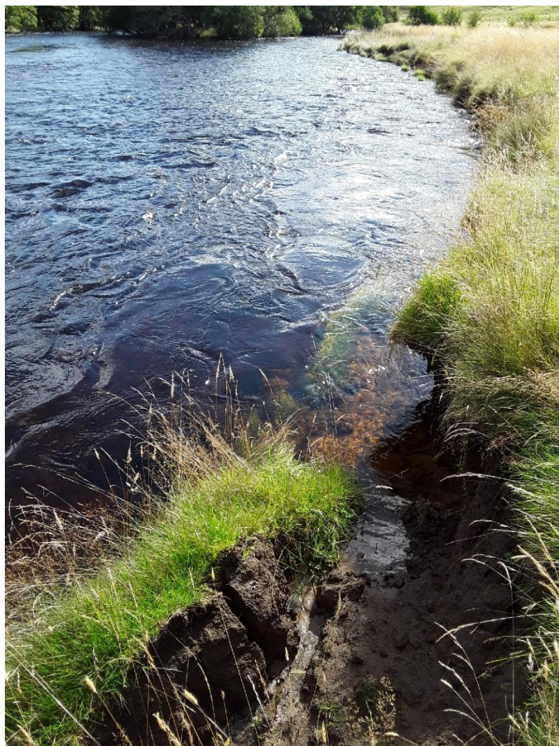
Photo 2: Example of erosion of the banks on the River Moriston
